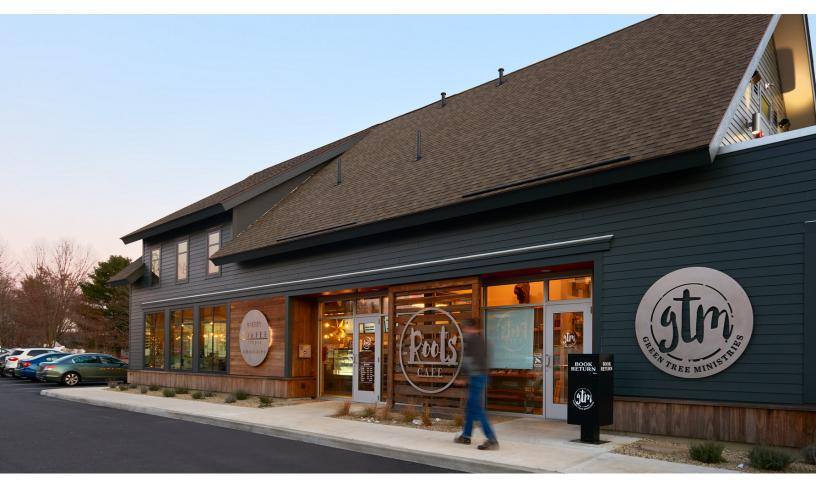
Roots Café, located in Westbrook, Maine, features an envelope comprising a mix of HardiePlank lap siding and Kebony Clear cladding.
