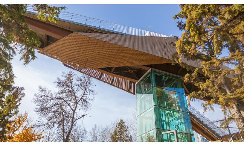
A boxlike, cable-mechanized, incline elevator, the funicular can transport mobility aids, bikes and strollers, and runs beside by a staircase for those who prefer to walk. It is located in downtown Edmonton.
